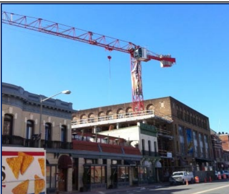
Figure 1: Tower Crane Located in Center of New Addition, Picture Courtesy of Luis Ortiz
